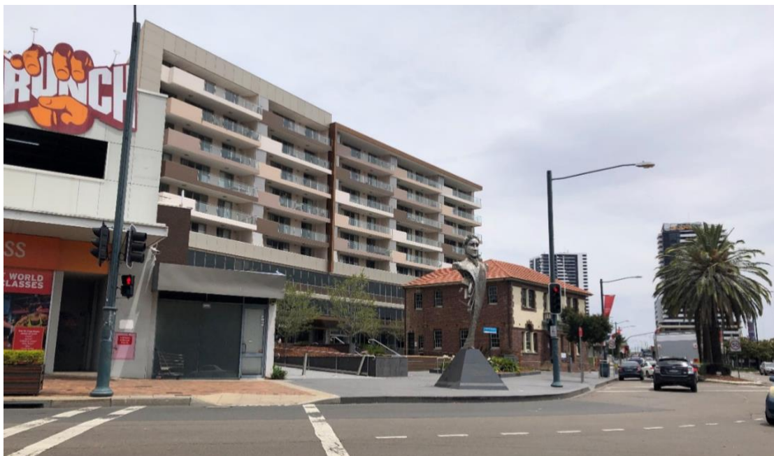
Figure 6: Photo looking south-west towards the 'Memorial School of Arts Building', Macquarie Monument and 'row of three palm trees', all of which are heritage items identified under LEP 2008. Source: Architectus
